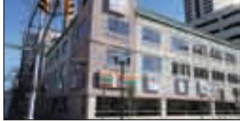
ATTENTION INVESTORS: AMAZING OPPORTUNITY 3-story commercial building next to Tropicana $4,900,000
